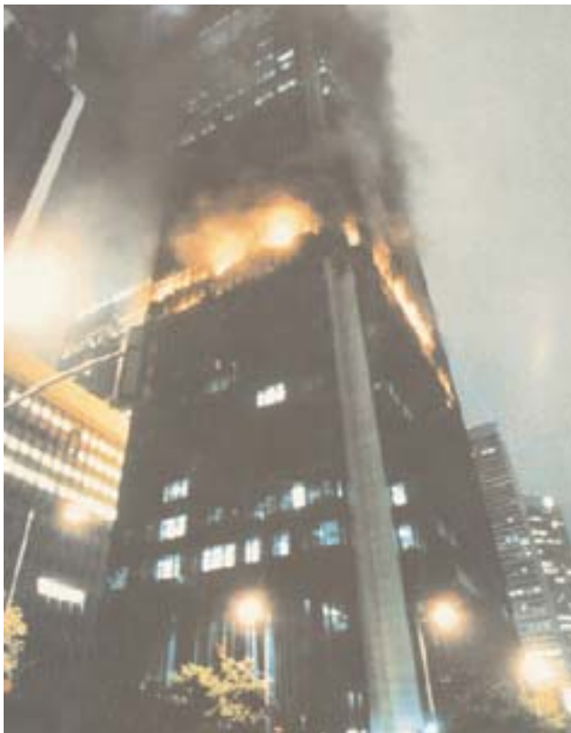
Fig. 6.3. First Interstate Bank in Los Angeles During May 4, 1988 Fire ( www.lafire.com )
